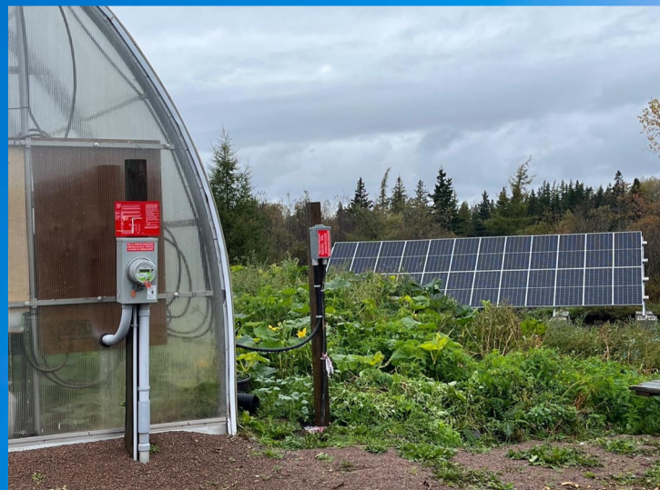
Solar schools project - solar array installations
