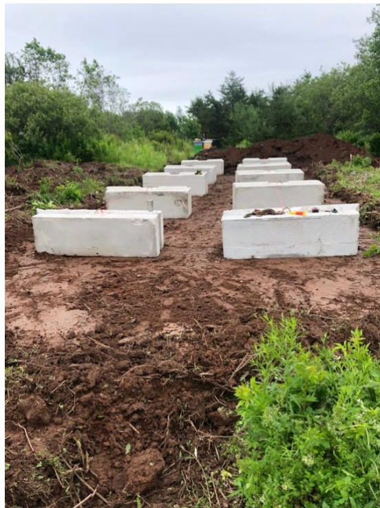
Concrete footings were installed in early July 2023 to mount the solar system at Port Elgin Regional School. Photo: Woody Thompson of Fundy Solar.
