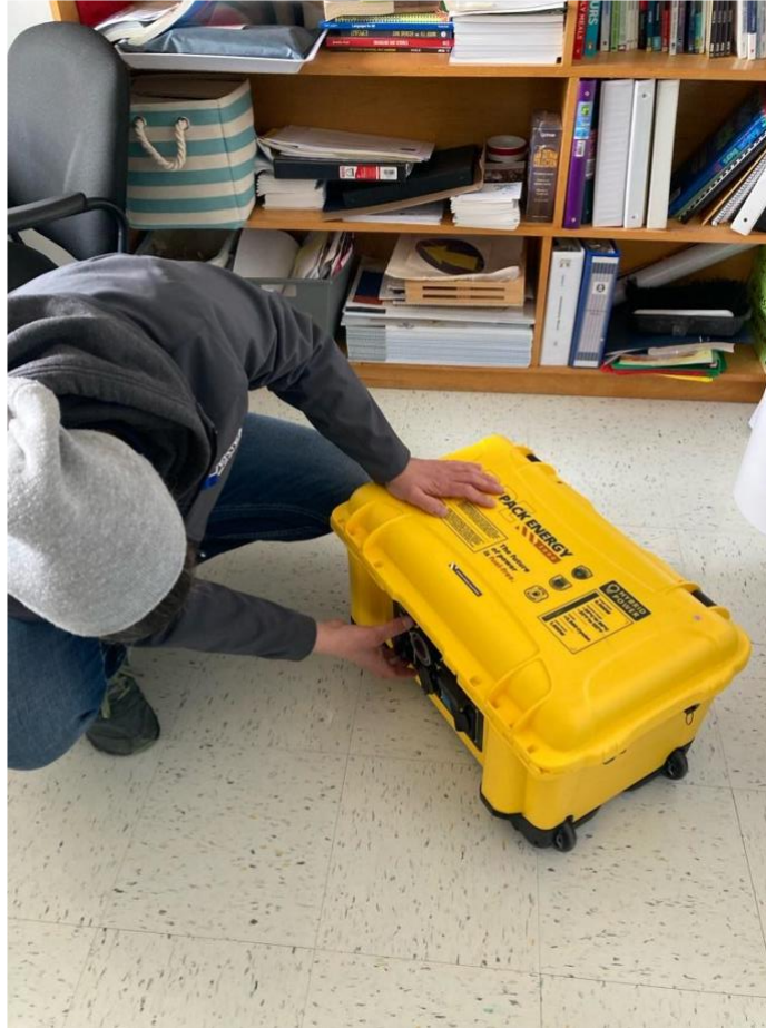
Annie, a solar installer from Vertex Solar Solutions, showing EOS and school staff how the battery pack works.
