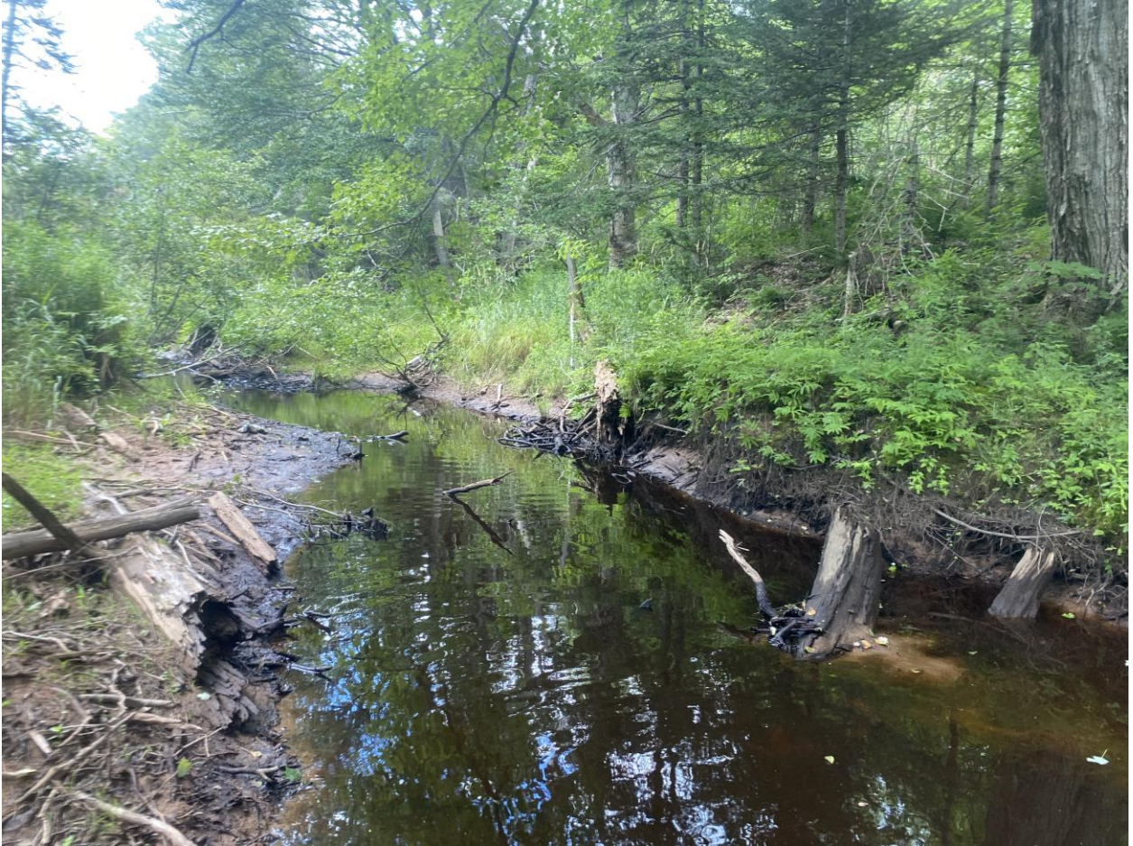
Figure 6: A picture of SB-21, showing eroded banks.
