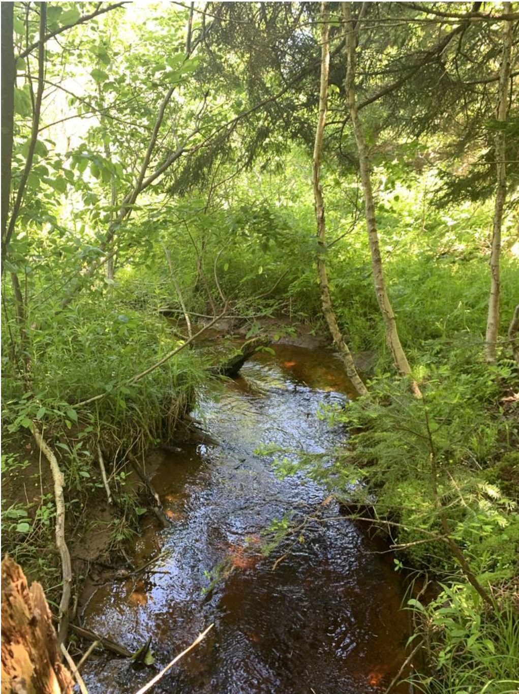
Figure 4: A photo of SB-04 showing a slightly eroded bank.
