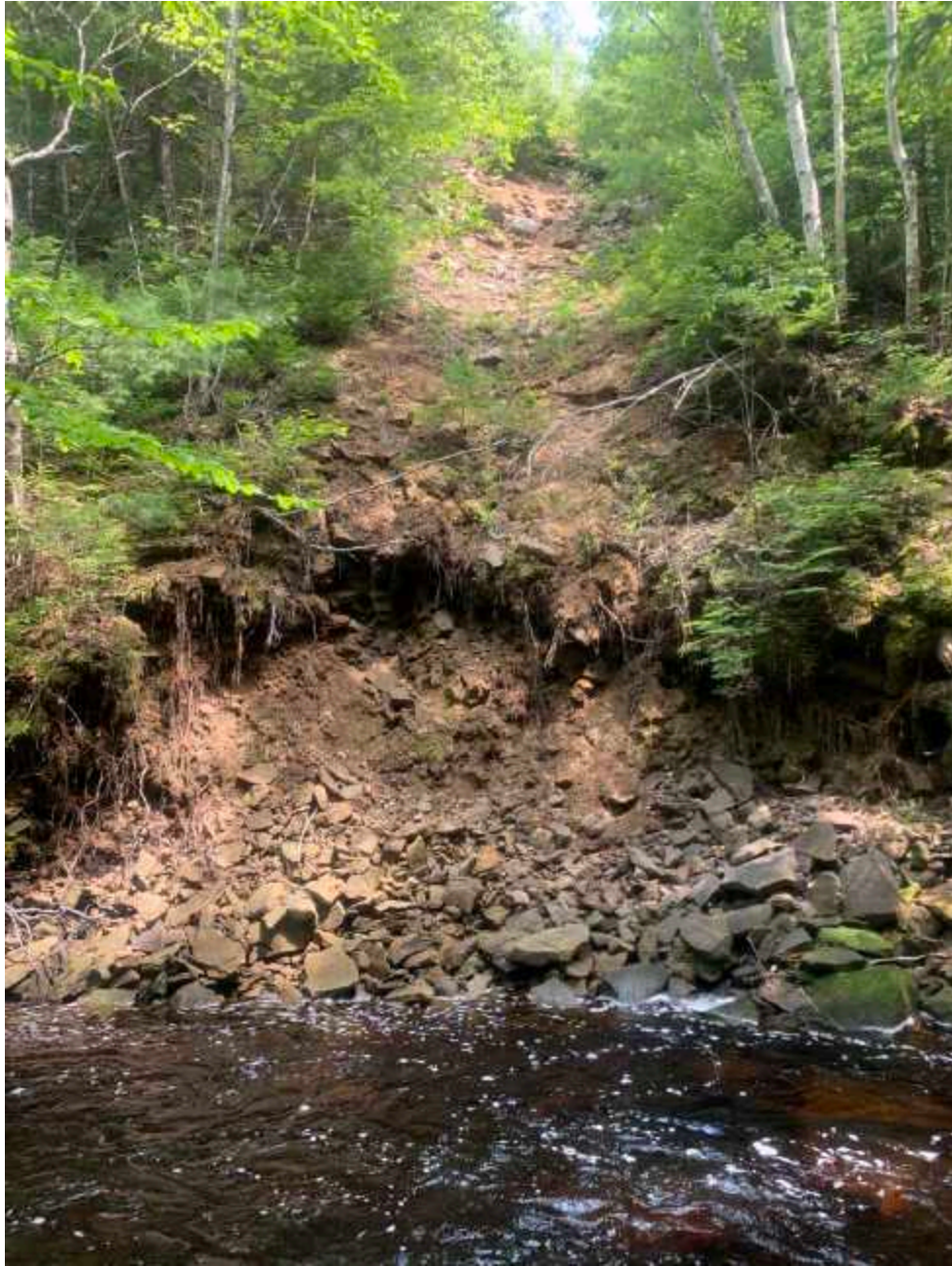
Figure 8: Photo from JB-57 showing a heavily eroded section of the bank
