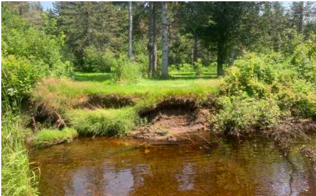
Figure 14: Photo of JB-70, showing an eroding bank, where a property owner has cut the grass right to the edge of the stream bank
