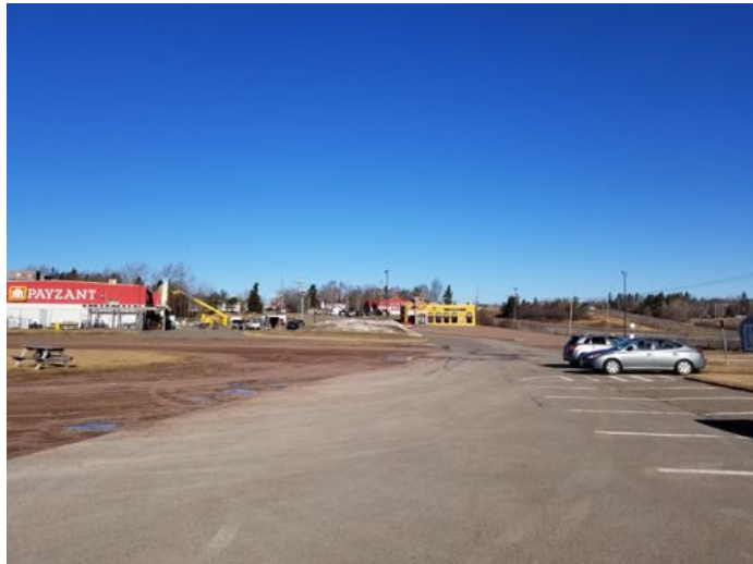
Looking up Mallard Drive from the parking space to be depaved. The parking area is in a lower lying area that receives runoff from further uphill.
