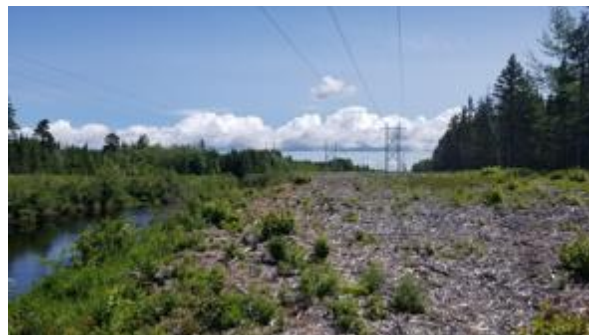
Figure 11: Powerline clearing off Route 15
