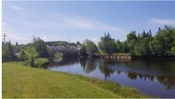
Figure 14: Wooden shore stabilization near the Main St. bridge in Port Elgin
