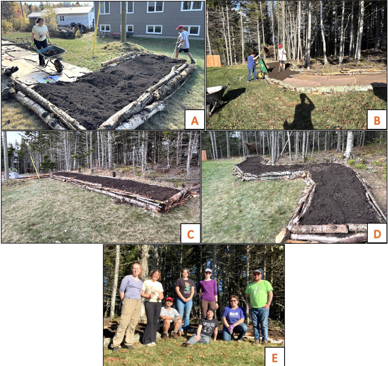
Figure 6: A through D – EOS staff and volunteers building up raised two natural beds for the new food forest at Amlamgog First Nation, and E – EOS staff, project partners, and volunteers helping to build the raised beds.
