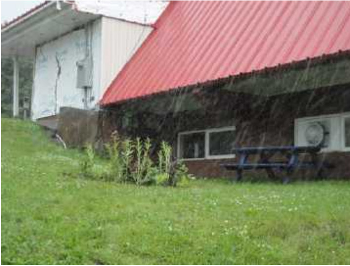
St. Ed's Hall, Dorchester rain garden catching rain off the roof
