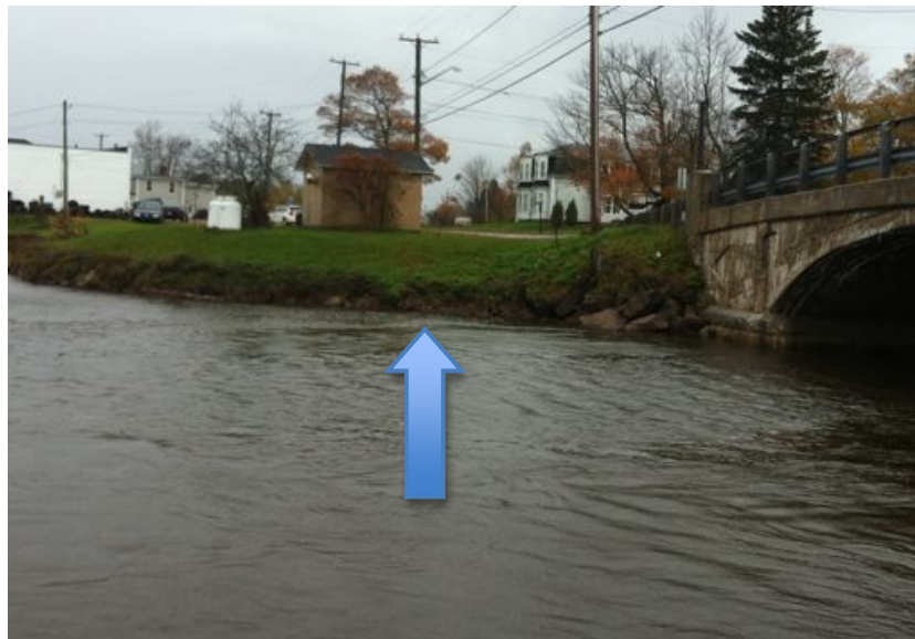
Erosion on the bank of the Gaspereau River below Main St. lift station. Photo: Anne Goodwin.
